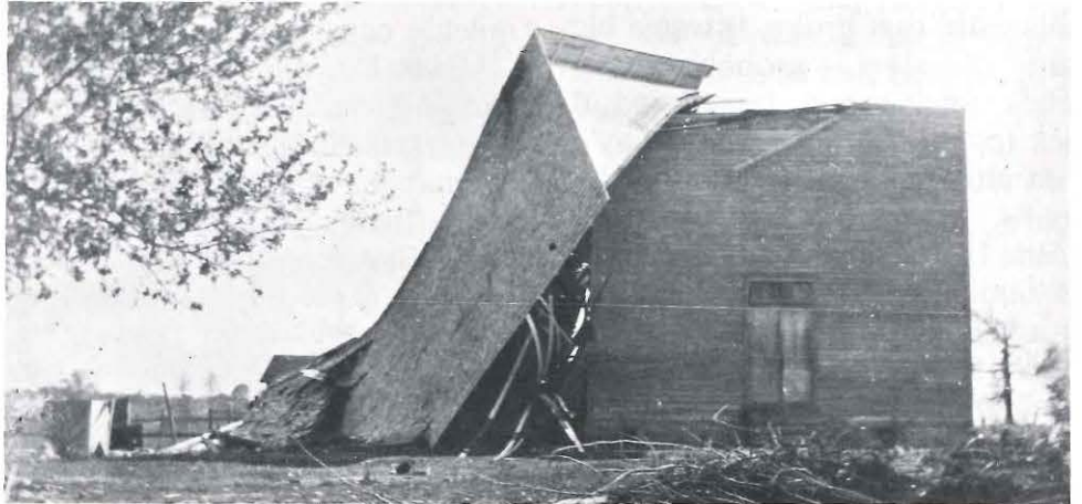
The church that was destroyed by a tornado in the 1920s.
