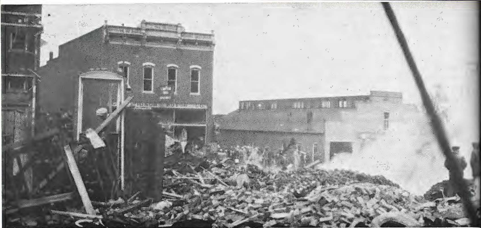
Looking toward the north side of East Main the day after the explosion.
