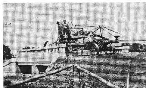
The three photos above were taken in 1922 while Highway 63 was being built.
