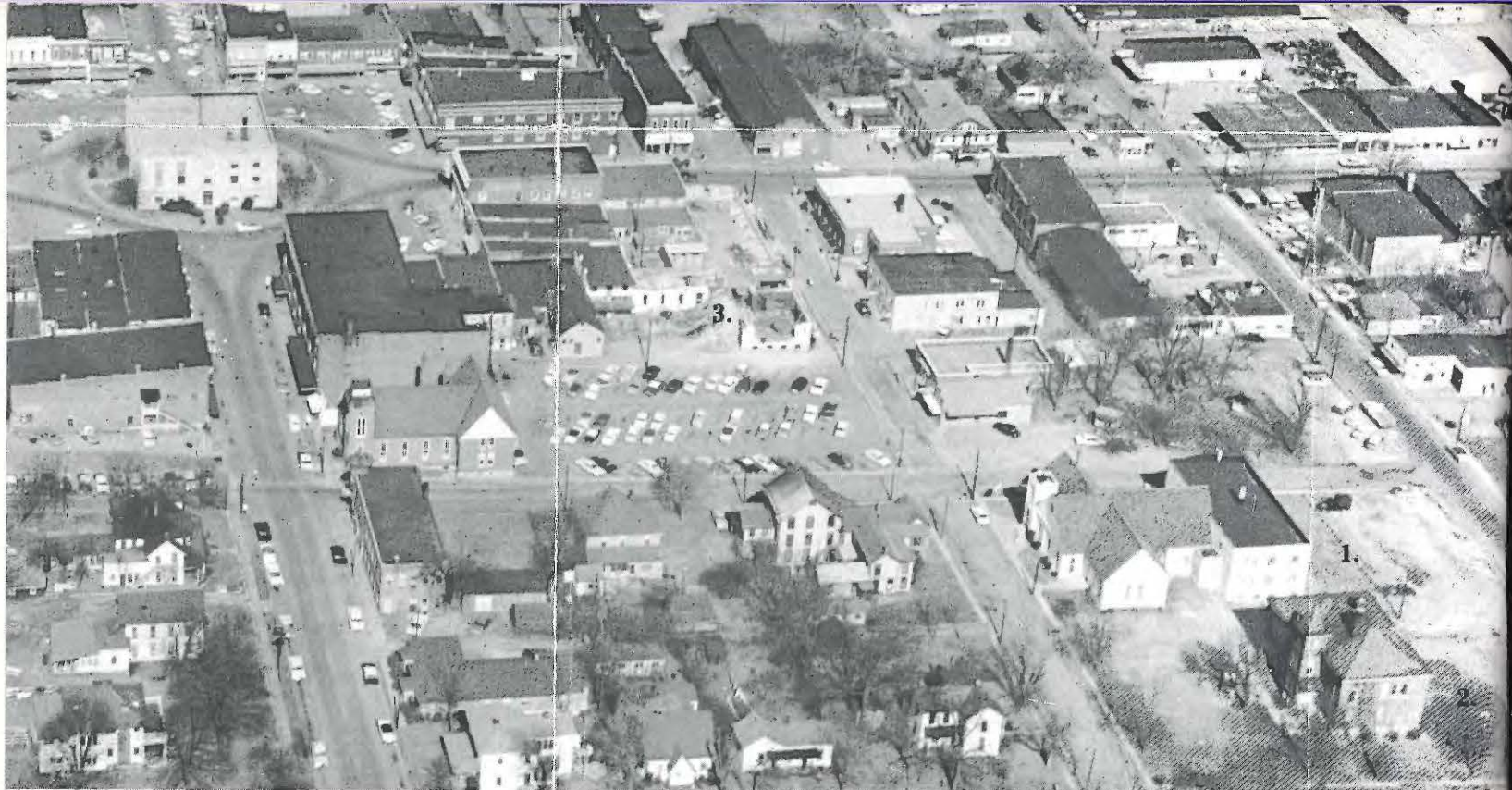
Aerial photo of West Plains. 1. The educational addition at First Baptist Church which housed Mo-Ark College. 2. Old Central High School. 3. Demolition site of Arcade Hotel. This photo originally appeared in Gazette number five dated 1948. It was actually taken several years later.
