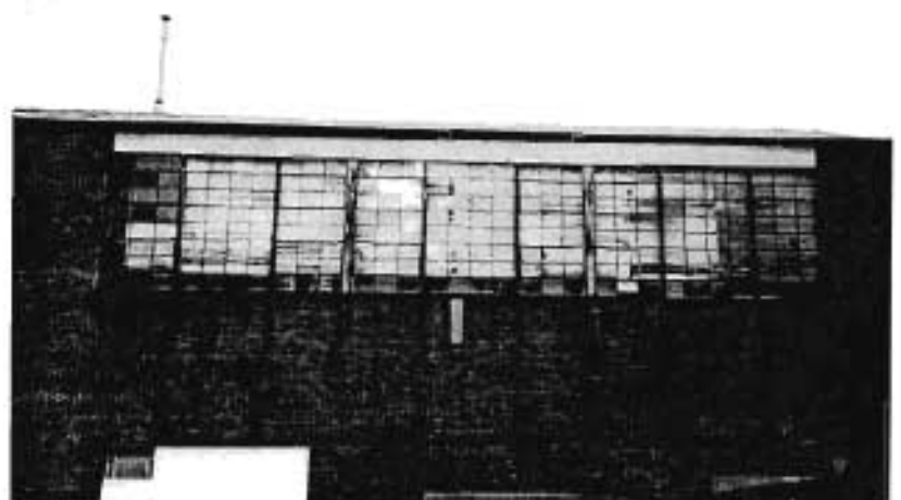
Douglass School Gymnasium View from west
