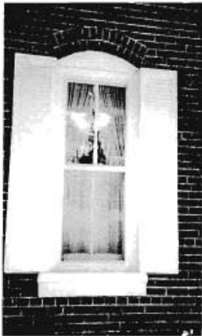
Douglass School Detail: original window on facade
