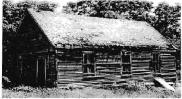
Lincoln School Nevada, MO. View from northwest
