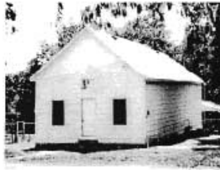
Douglass School Butler, MO. View from northeast
