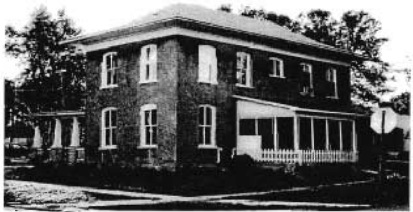
Western Baptist Bible College, Dormitory Macon, MO View from southeast
