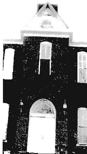
Lincoln School View from east: central projecting bay
