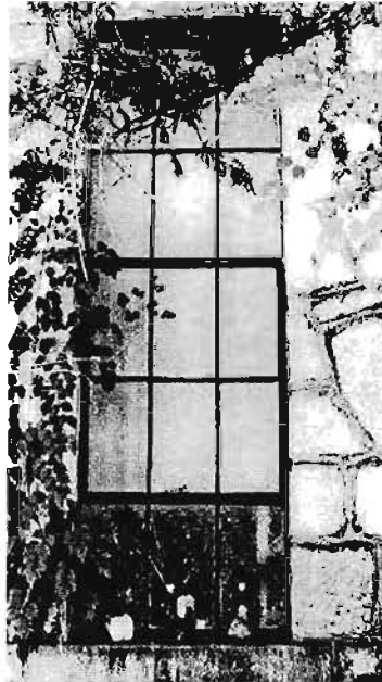
Lincoln School Detail: original casement window and stone masonry
