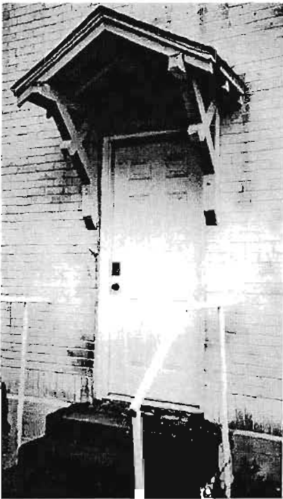
Crispus Attucks School Detail: entrance with gabled awning
