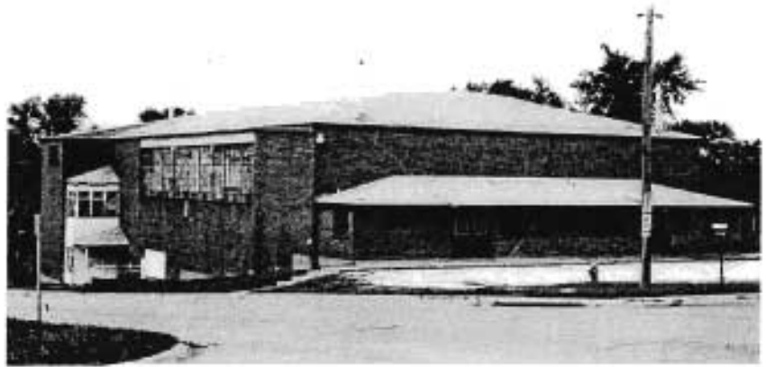
Douglass School Gymnasium Festus, MO. View from southwest
