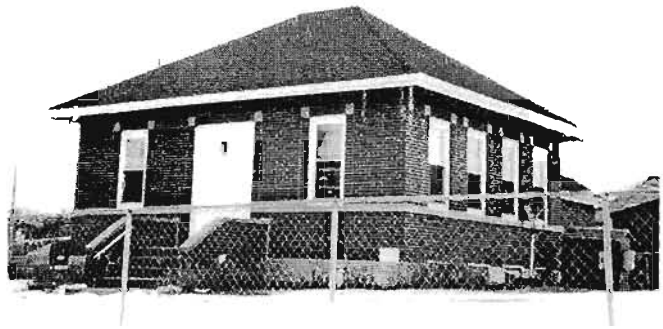
Garfield School Trenton, MO. View from southwest
