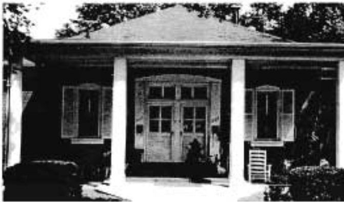
Douglass School View from south: facade
