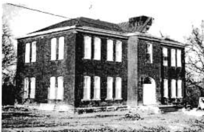
Lincoln School Clinton, MO. View from southeast
