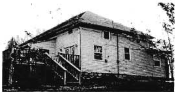
Franklin School View from northeast
