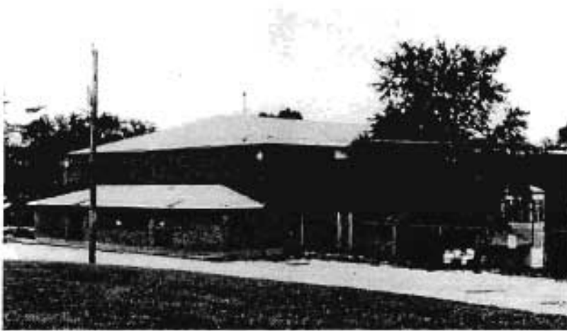
Douglass School Gymnasium View from southeast
