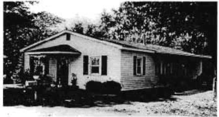
Lincoln School St. Mary, MO. View from north
