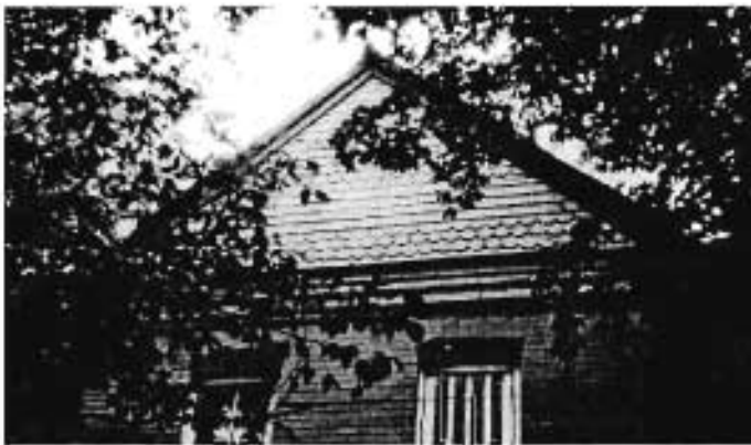
Langston School View from northeast: detail of gable
