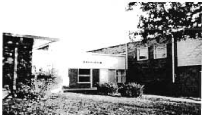
Garrison School View from northwest: facade
