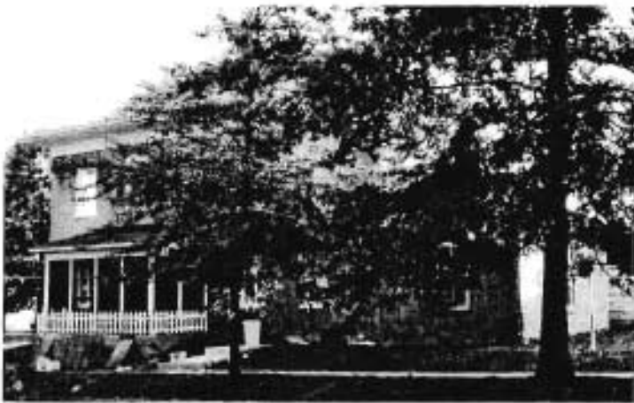
Western Baptist Bible College, Dormitory View from northeast
