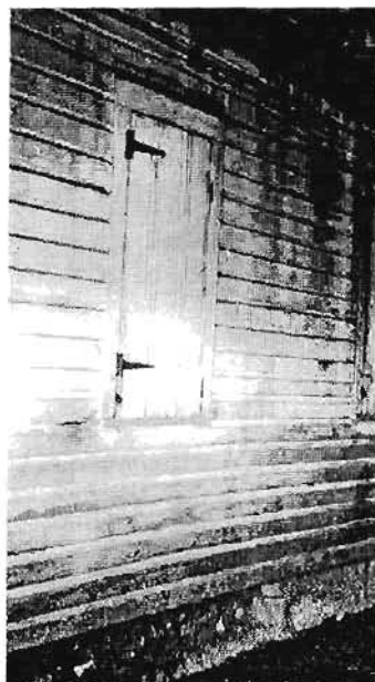
Tebo School Original shutters on eastern exterior wall
