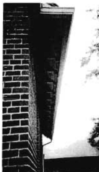
Lincoln School Eaves, rafter tails
