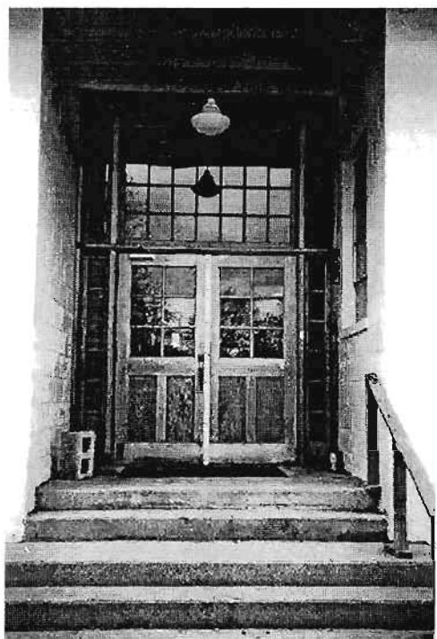
Park School View from east: entrance
