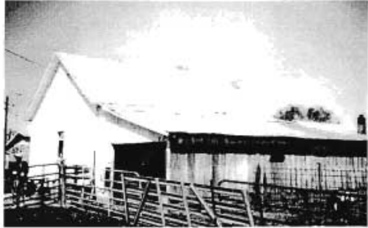
Tebo School Vcn., Leeton, MO View from southeast
