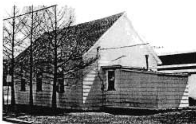
Bryant AME Chapel View from northwest
