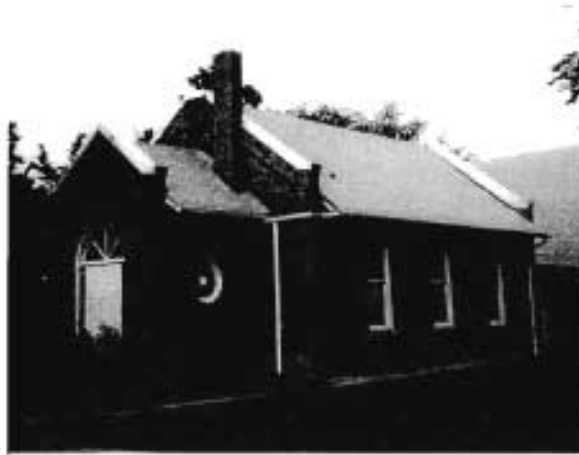
Lincoln School Rolla, MO. View from southwest
