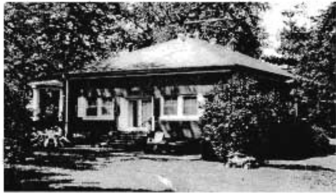
Douglass School View from east
